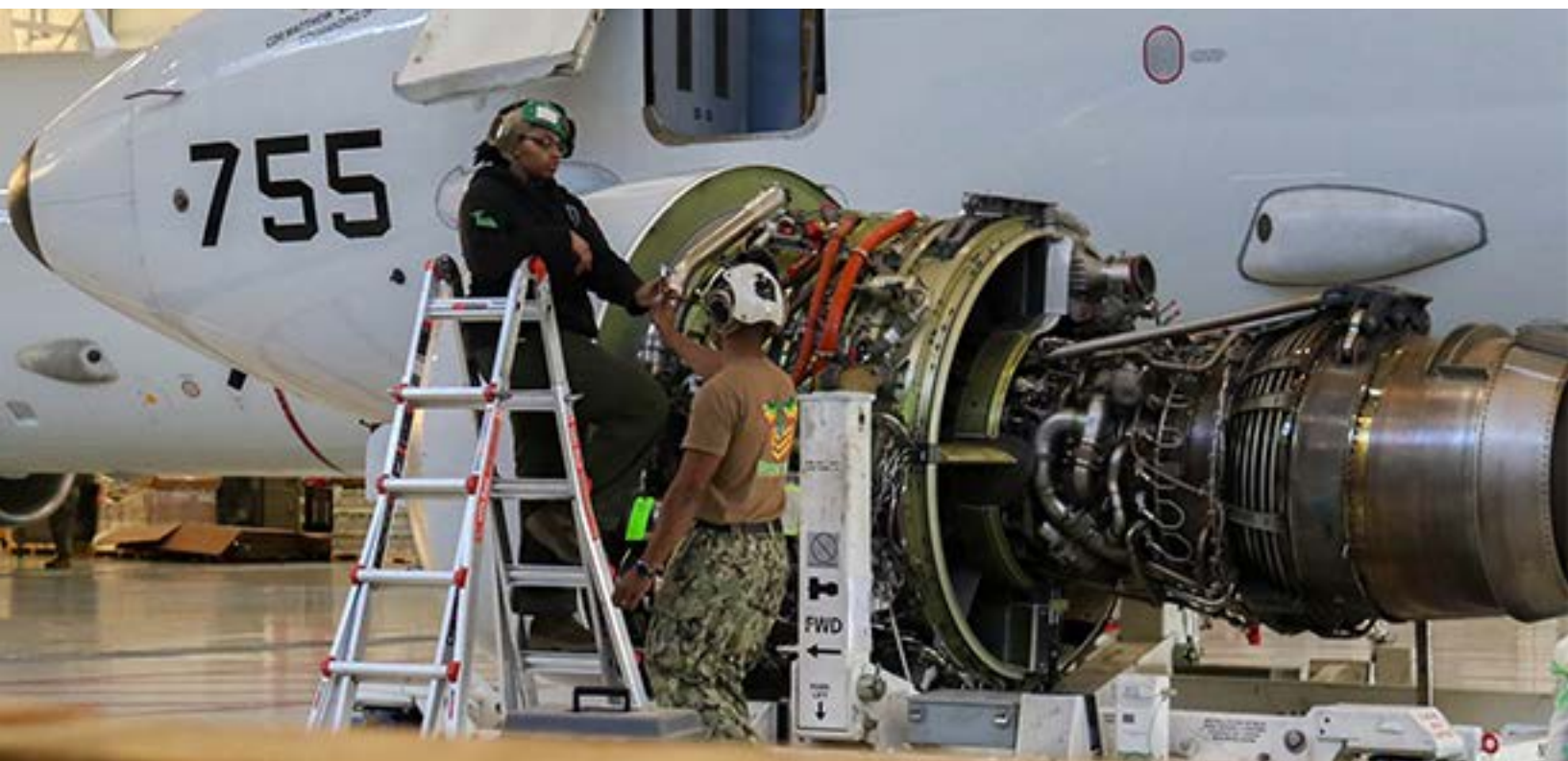
(LEFT & BELOW) WHIDBEY ISLAND, Wash. (Nov. 16, 2023) Our aircraft work hard, but VP-4's maintenance team works harder. Their dedication to safety and operational excellence means they can replace an entire engine with both efficiency and meticulous attention to detail. This evolution underscores their unwavering commitment to upholding the highest standards in aircraft maintenance. Photo courtesy of VP-4.
