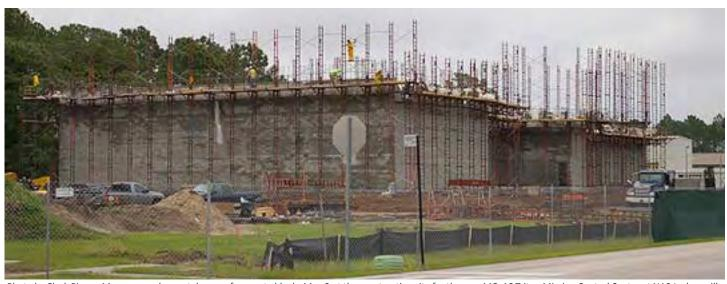
Photo by Clark Pierce. Masonry workers set dozens of concrete blocks May 2 at the construction site for the new MQ-4C Triton Mission Control Center at NAS Jacksonville.
