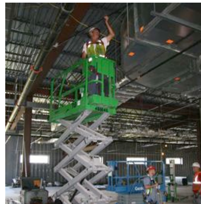
Photo by Clark Pierce. (At left) A technician checks his measurements for air-conditioning ducts in the new P-8A Poseidon schoolhouse for maintainers.
